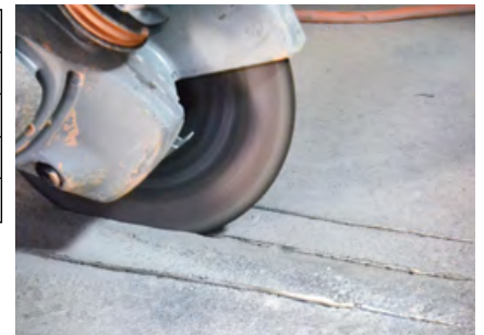
Creation of traces on reinforced concrete.
